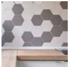
DADO CERAMIC TILES 600 MM ABOVE THE COUNTER
