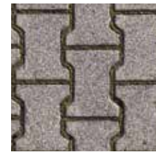
INTERNAL ROADS INTERLOCKING BLOCKS/ TREMIX CONCRETE ROAD
