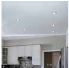
WALL / CEILING OIL BOUND DISTEMPER
