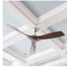
CEILING OIL BOUND DISTEMPER
