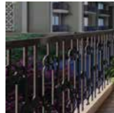
RAILING WROUGHT IRON RAILING
