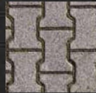
INTERNAL ROADS INTERLOCKING BLOCKS/ TREMIX CONCRETE ROAD
