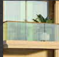
RAILING GLASS/SS RAILING
